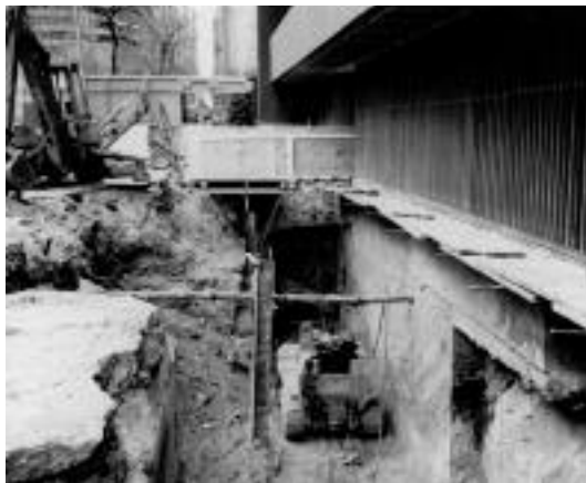
Construction in 1992 during the Society's $10.5 million expansion. Photo © Jeff Nemeth.
